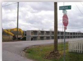
Bamore Road Reconstruction Project
