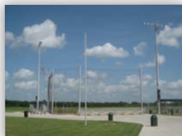
Seabourne Creek Regional Sports Complex Lighting
